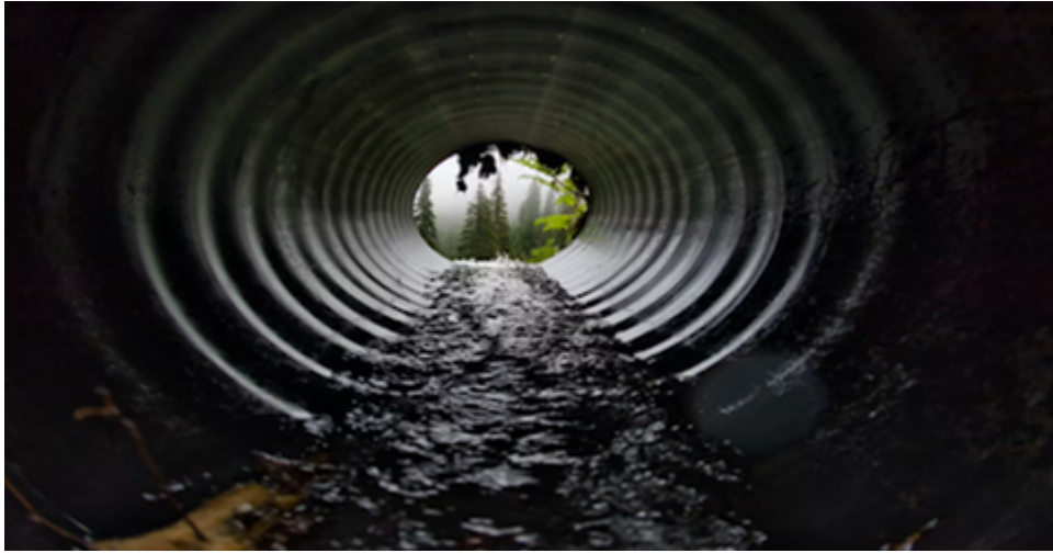
Image: Sewer outlet (end of pipe solutions)
